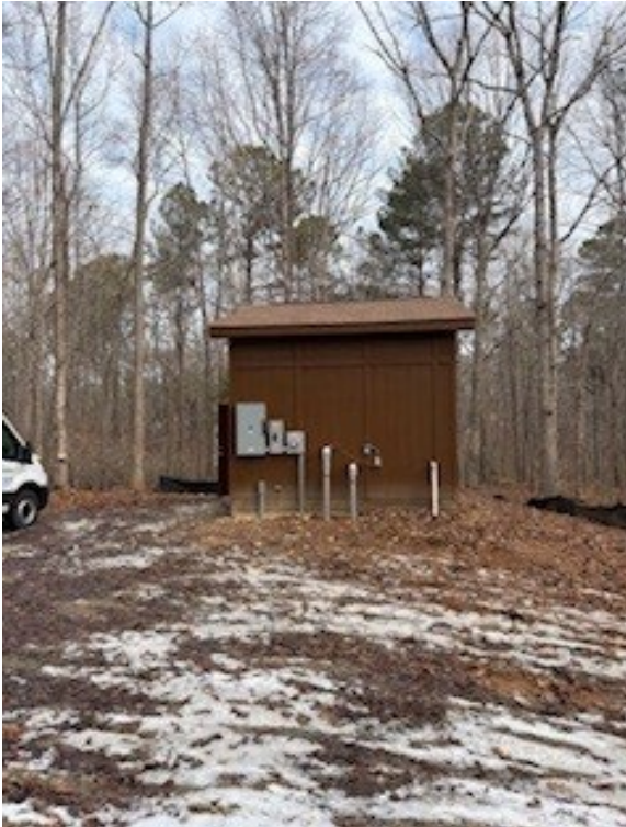
Figure 4 Old Mill Trace Well House
