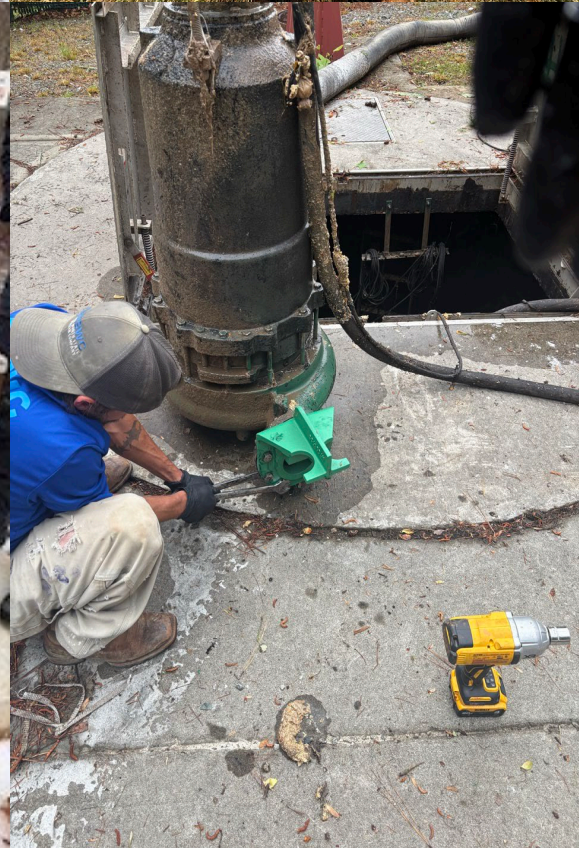
Figure 7 Repairs at Lift Station A Briar Chapel
